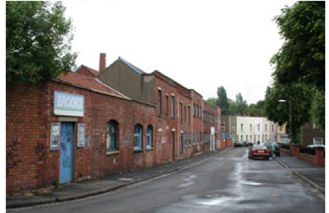
Morley St brick built workshops
